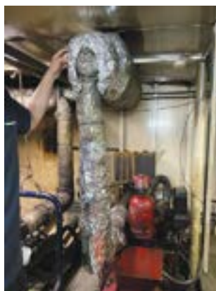
Aluminium foil is not appropriate lagging
